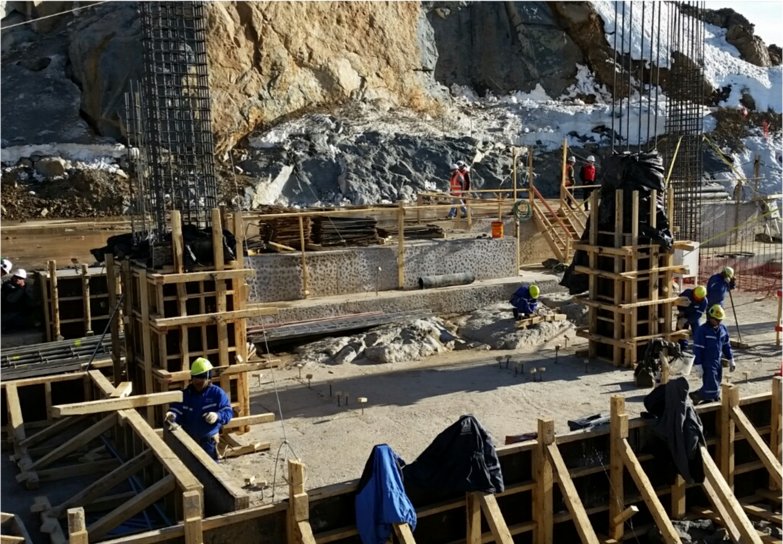
LSST Construction – Above Ground on Pachón!
